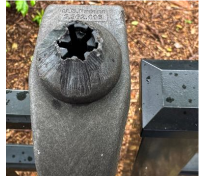
Most likely the shaft is damaged, so Option B
